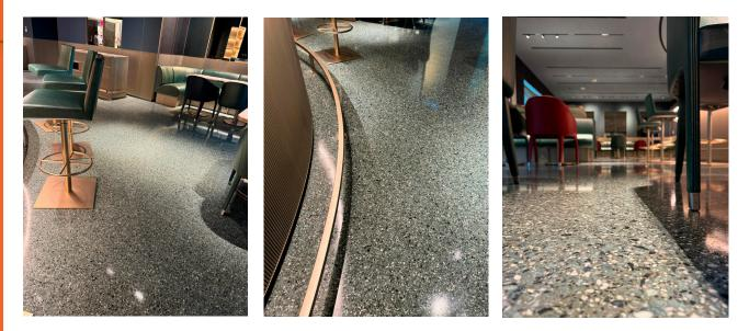
The substrates were initially primed with **Strongcoat UN101**; Subsequently, the resin was blended with the aggregates. Once the mixing process was complete, the mixed **Strongcoat Terrazzo** mortar was applied to the primed surface and compacted to achieve the desired thickness.
